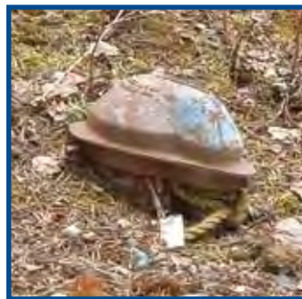
Figure 1. Well casing stick up less than 30 cm (12 inches) from the ground surface
