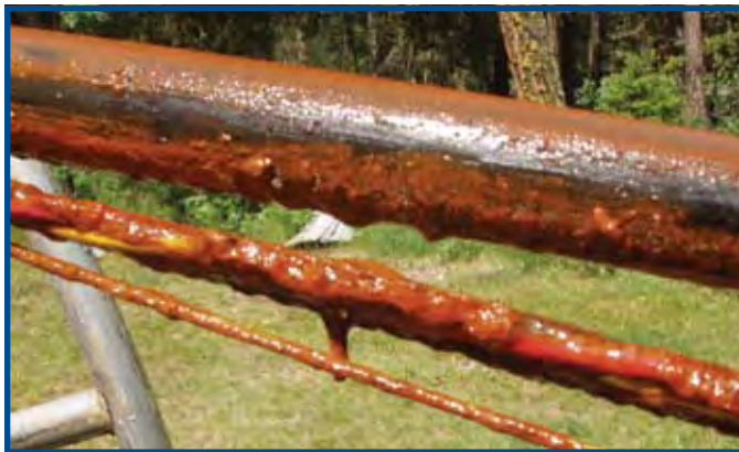
Figure 3. Biofilm on well wiring
