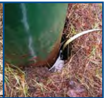
Figure 2. Well with gap between casing and ground – no surface seal
